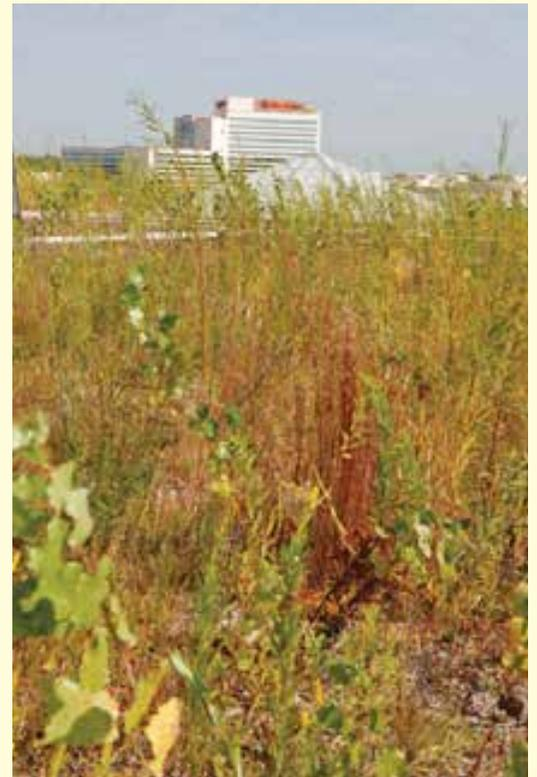
▶ Green roofs are another storm water treatment method which replicates natural processes by absorbing rain fall and returning it to the atmosphere through evaporation and transpiration.
